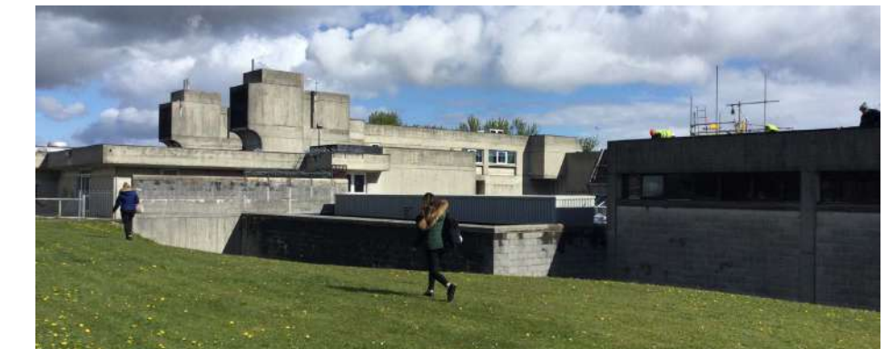
4 - View towards main building from the South
