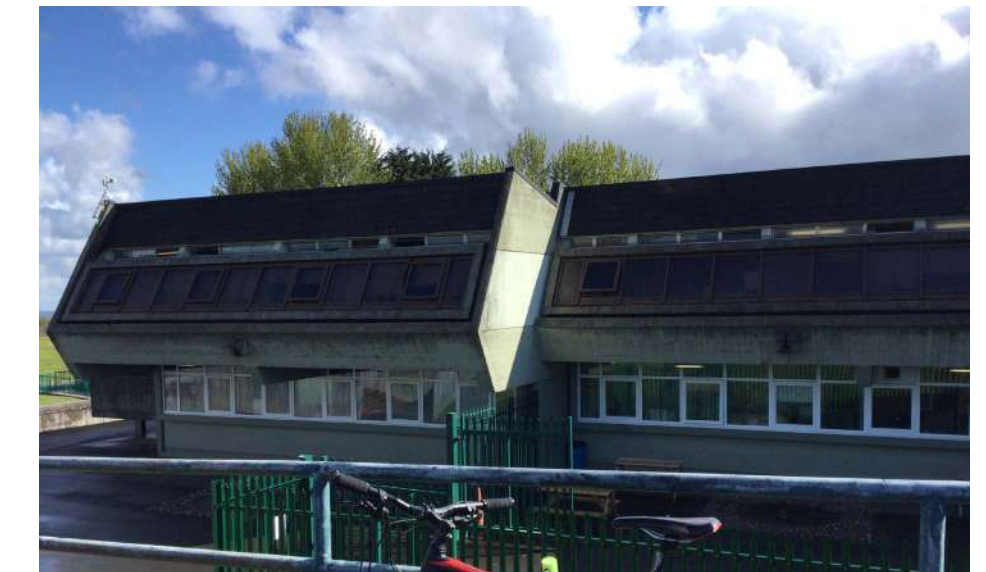
5 - View towards one of the original "Brutalist" teaching blocks
