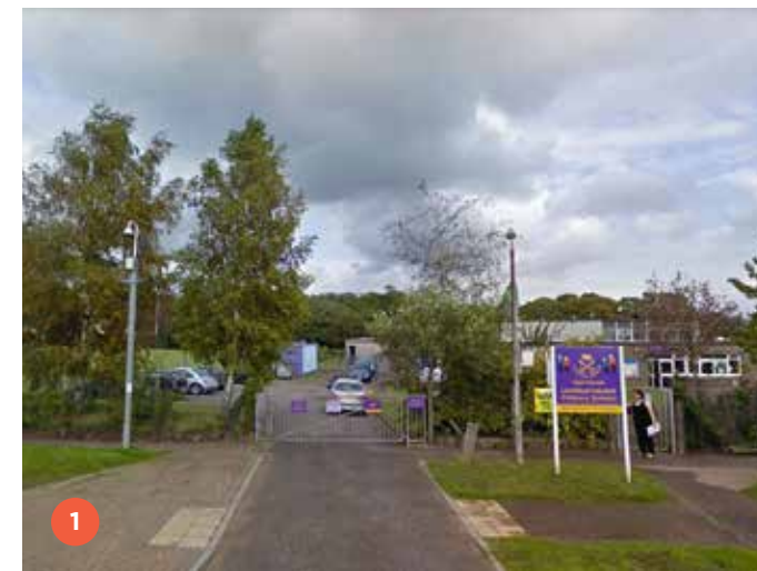
View towards current main entrance
