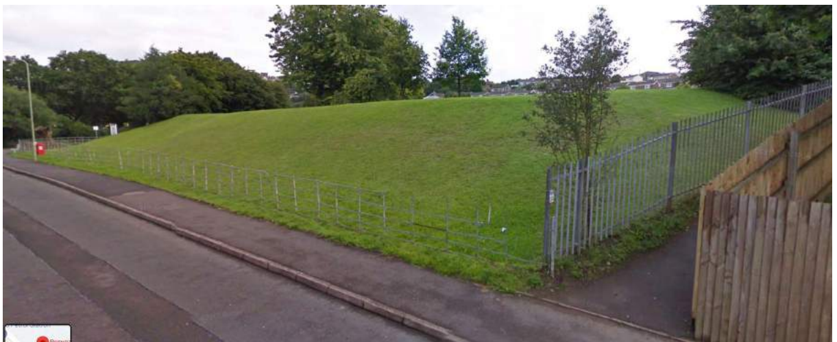
Figure 4: Embankment in Flood Zone B
