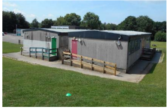
Photograph 8. Buildings B2 and B3, cabin style structures.
