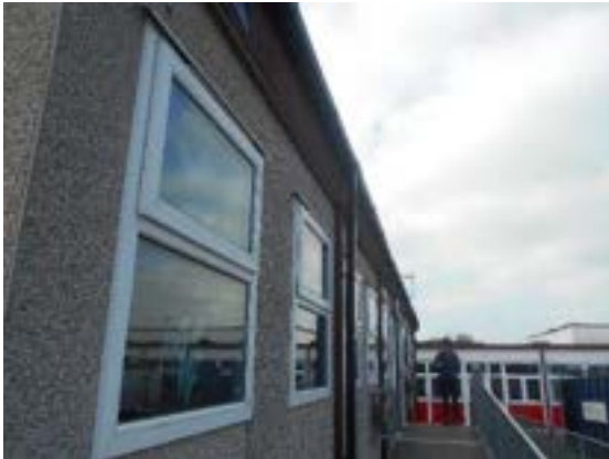
Photograph 3. Building B2 - north-west elevation with B3 beyond.
