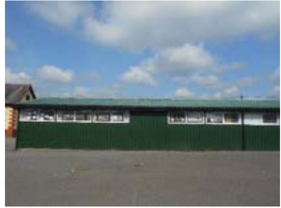
Photograph 8. Building B6 corrugated metal contained cabin, with corrugated roof
