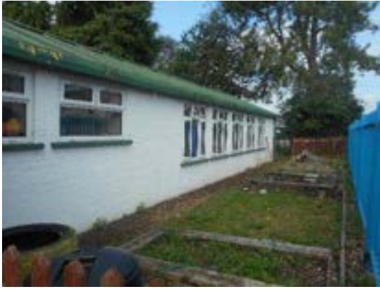
Photograph 1. Northern aspect of Building B1 and adjacent grassland.
